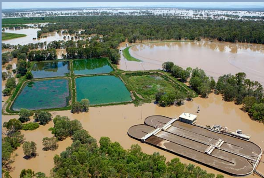
Floodwaters surround the Rockhampton STP. Photo Janie Barratt
