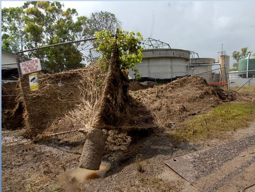
Dalby Water Treatment Plant after 2011 Floods
